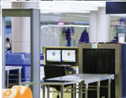
Airport Security Checkpoint, Luggage X-Ray Scanner, Gate Control System
